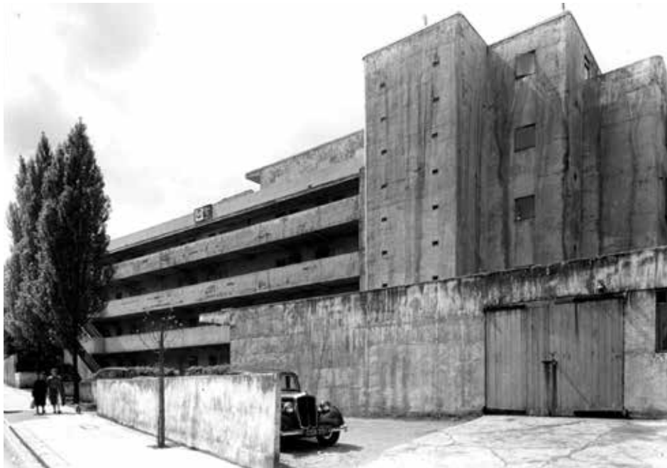
Fig. 13 – Designed by Wells Coates for Jack and Molly Pritchard, the Isokon Building opened in 1934 as a progressive experiment in new ways of urban living. It was the first block ever to be built chiefly using reinforced concrete. It was painted brown to avoid being bombed during the war.
